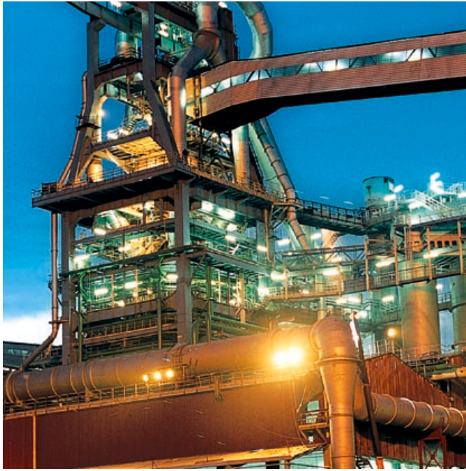
Industrial application: Refinery
