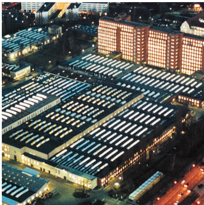
Switchgear Factory in Berlin, Germany
